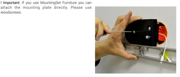
Step 2 ! Optional: The mounting plate provides an additional mounting hole on the left side. It is located outside the box directly on the wall and gives free additional stability if necessary.
